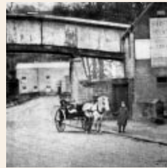
c Footbridge between Milford Mill buildings The main road was formerly crossed by an overhead gangway, linking the two parts of the Mill complex. Parts of its supports can still be seen in the roadside wall of the surviving Dyehouse. It was taken down in the late 1930s, as it had become an obstruction to double-decker buses.
