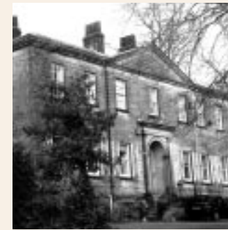
e Milford House Now a residential and nursing home for the elderly, Milford House stands by the main road a short distance south of here. It was built in 1792 for Jedediah Strutt. Designed in a style reflecting his new status, it overlooked the mills which steadily increased his wealth.
