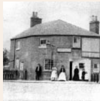
f Tollbar Cottage, about 1870 This toll-house collected charges for use of the bridge and turnpike roads. The bridge was widened in 1906 to provide space for pavements, and the toll-house was partly demolished. Its remains can be seen down beside the far end of the bridge.
