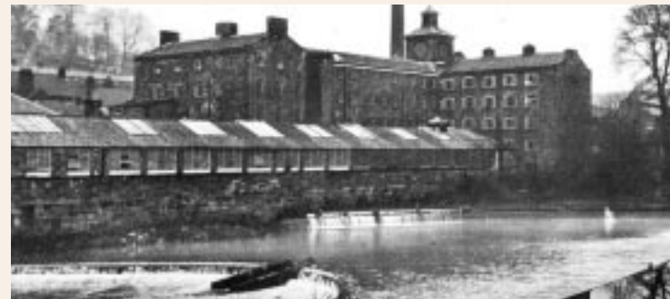
g Mill & Weirs, Milford, looking north towards the bridge This part of the Milford Mill complex was built during the late 18th and early 19th centuries. It stood until 1964 behind the Strutt Arms Hotel, on land now partly occupied by the Mill House public house. It was powered by water from the Derwent channelled into a goyt. The wheel-pits may still be seen near the Mill House. The bell above the goyt, beside the Dyehouse, once hung in the Mill clock-tower.
